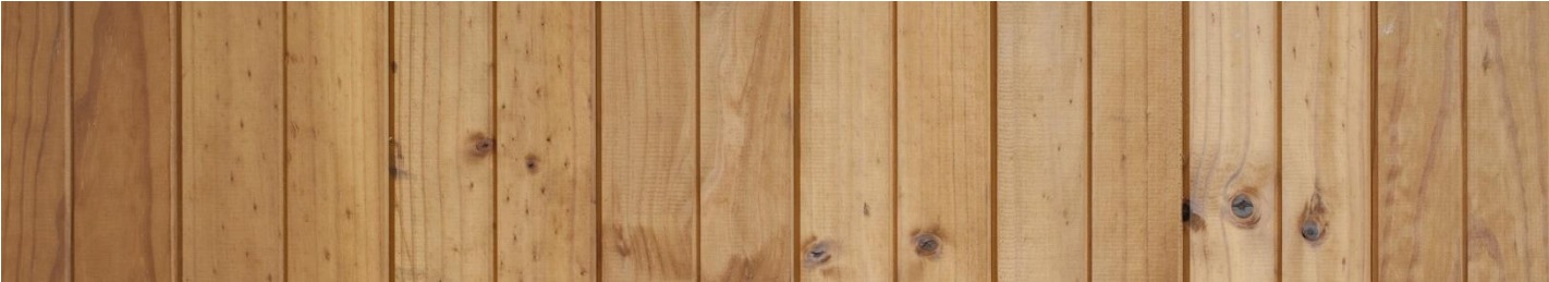
Detail of vertical boards
