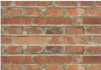
Brick wall detail
